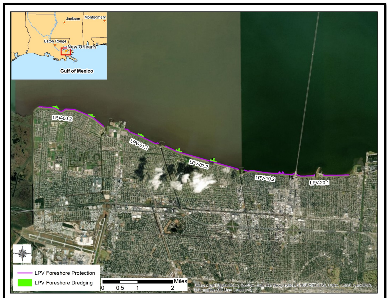
Figure 4. Foreshore protection placement and construction access dredging areas.
